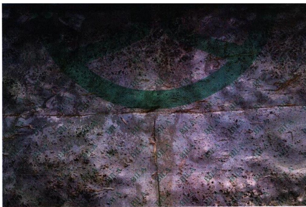
Photo 4 The T-shape joint after test
